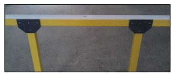
A removable HD Plastic strip was added to the top of the railing for added protection for the railing.
