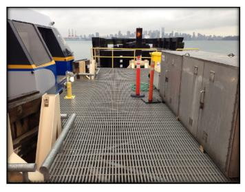
The maintenance dock at **Vancouver Seabus Terminal** was resurfaced with T-5000 2" Pultruded grating supplied by Fiberman.
